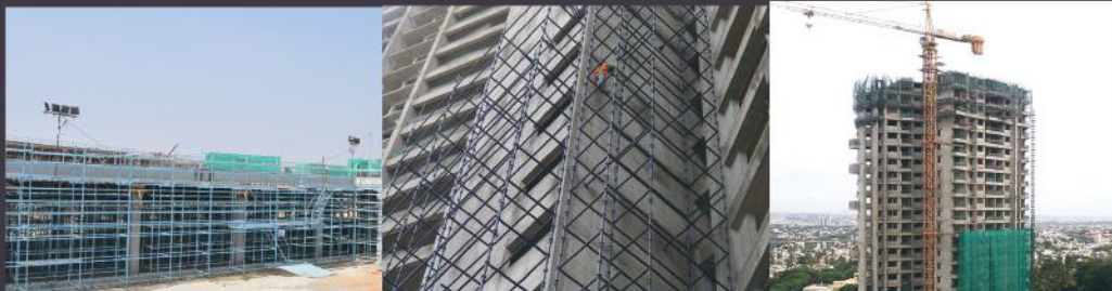
GSK PROJECT, SHIMIZU
